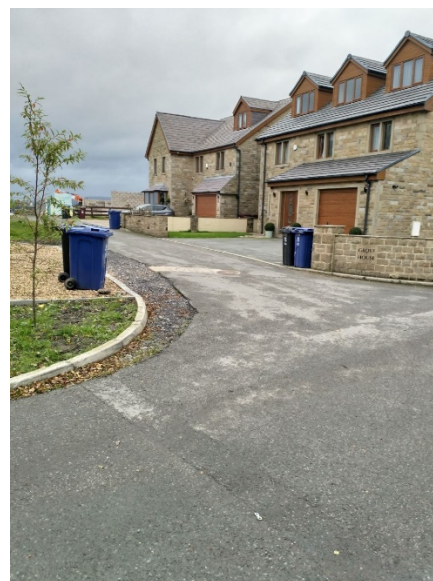
Photo showing the new kerb
