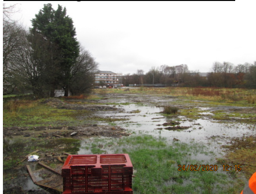
Site looking towards Barden Lane
