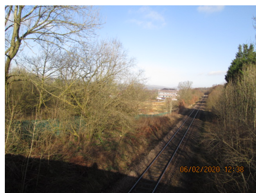
Railway to east boundary of the site
